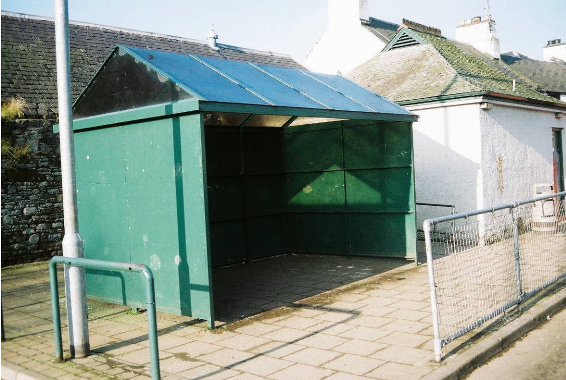
Figure LL: Bus Shelter in Earlston
