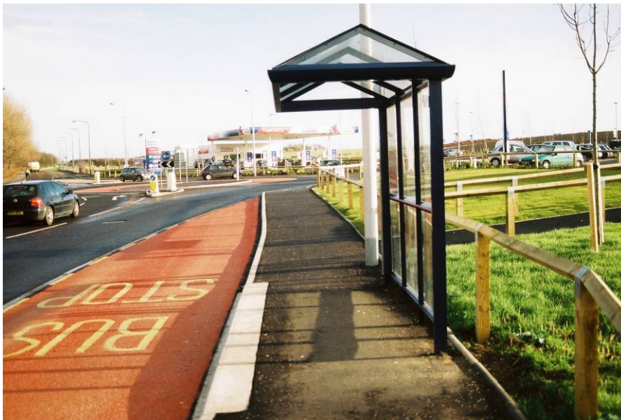
Figure PP: Bus shelter at North Berwick, Tesco store
