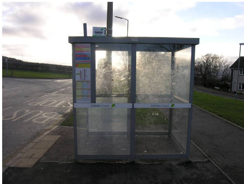
Figure BBB: Vandalised bus stop in Mayfield
