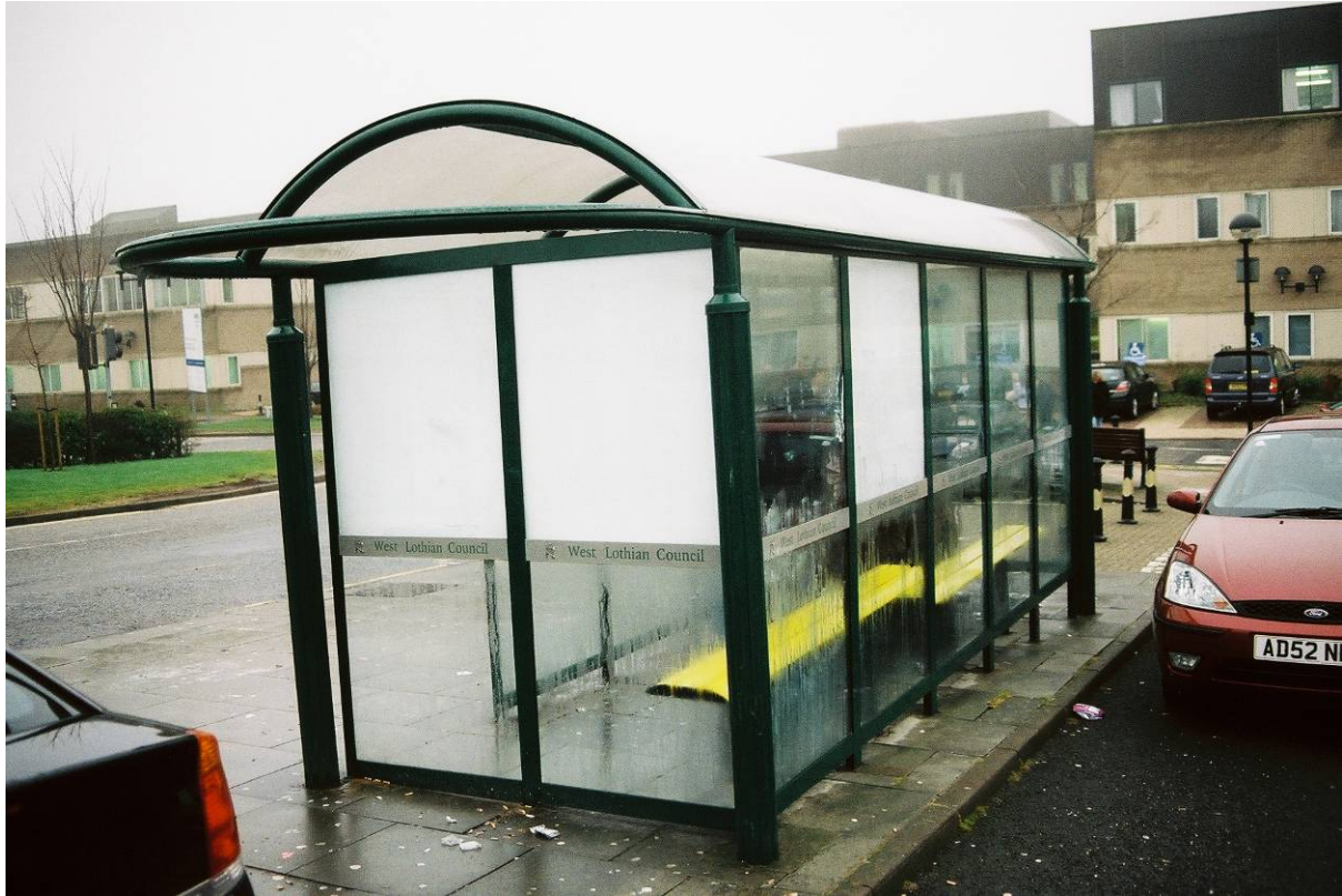
Figure YY: West Lothian Council bus shelter in Livingston
