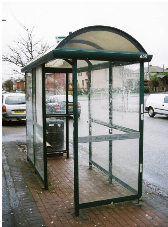
Figure SS: Vandalised shelter in Armadale, West Lothian
