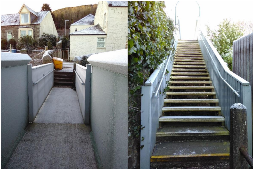
Figure 20. Footbridge at Hill Road Site
