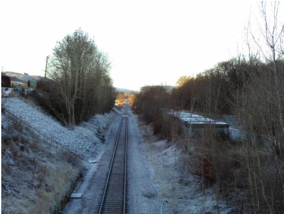
Figure 17. Former Station Site at West End of Newburgh
