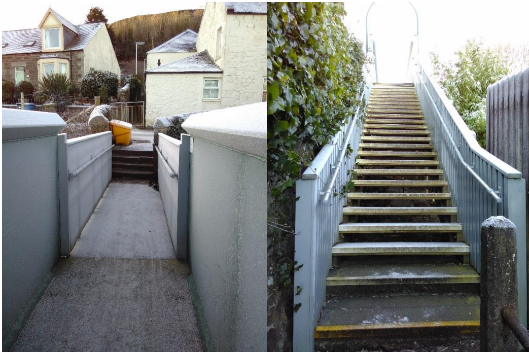
Figure 20. Footbridge at Hill Road Site
