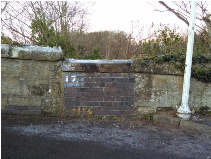
Figure 18. Former Access to West Site from Hill Road
